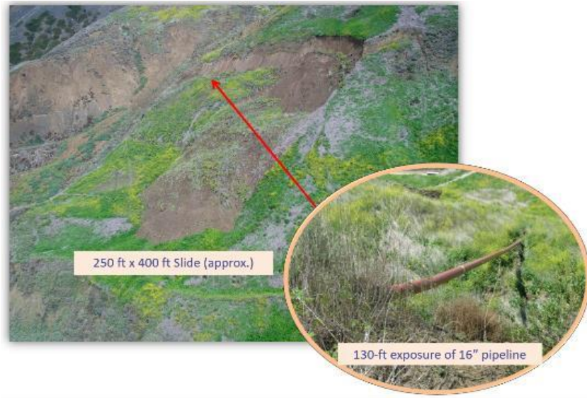
Figure 4. Pipeline Exposed by Pulling Up Through Soil in a Slide Zone
